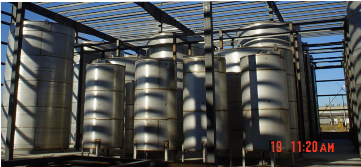
30,000 Gallon double walled and insulated storage tank with pumping, metering and remote control system
